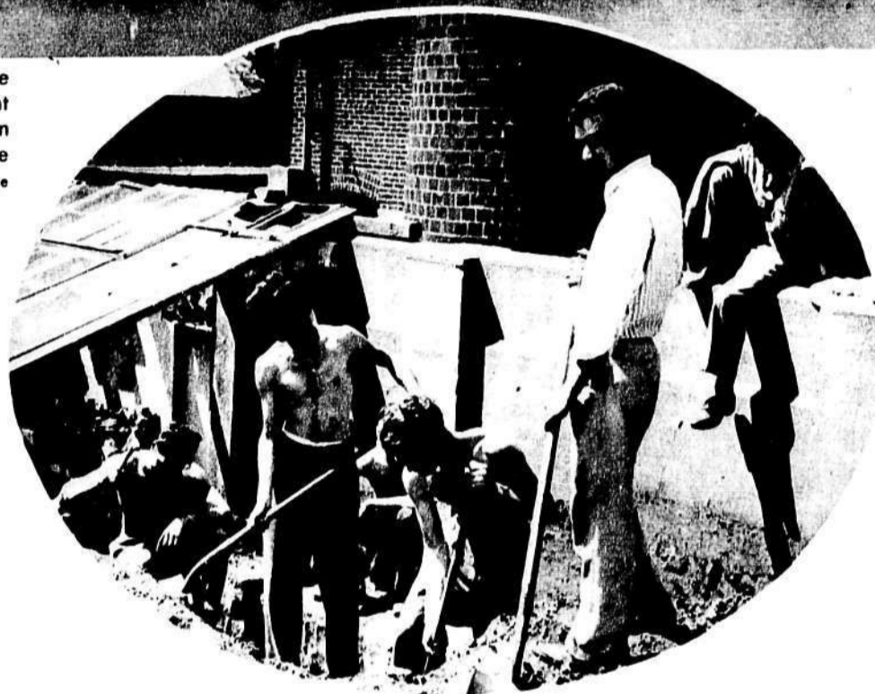
Looking Ahead — This construction gang is part of a botany class at Washington College, Chestertown, Md., making an enlargement to the greenhouse as part of their class project. Such work provides good training for the military job that is ahead of the boys.
