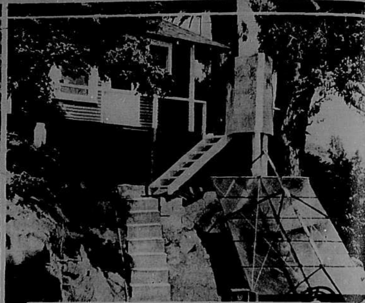
SUN BAKES BREAD with this apparatus perfected by Dr. C. G. Abbot at Mt. Wilson, Calif. It is called a solar stove, and was developed for the Smithsonian Institute. WIDE WORLD PHOTO
