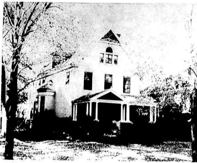
Above is a picture of the new Sigma Lambda Sigma house located at 155 South Lake Avenue. The house will accommodate approximately twenty-five members. Occupancy has been delayed because of lack of steel to complete the required fire escapes. The members of the house now living at the barracks expect to move into the new residence before the end of the month.
