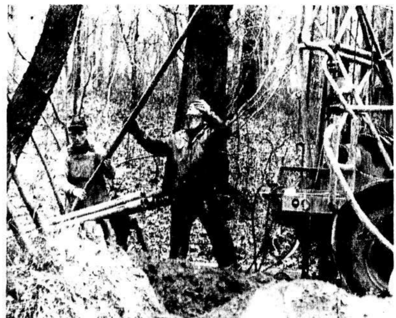
Hoisting a section of pipe to be fitted into drilling rig.
