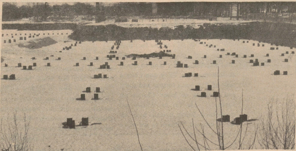
In 1965 plans were first made for a new Albany High to be completed by 1969. Today the pilings are in the ground and the last scheduled date of completion given was September, 1973. Because of the extraordinarily high projected costs (which are not feasible due to the limits of the city's borrowing power) the entire project is under study. There is some doubt as to how large a school is needed. This results from the precarious financial position of the city Catholic's high schools.
