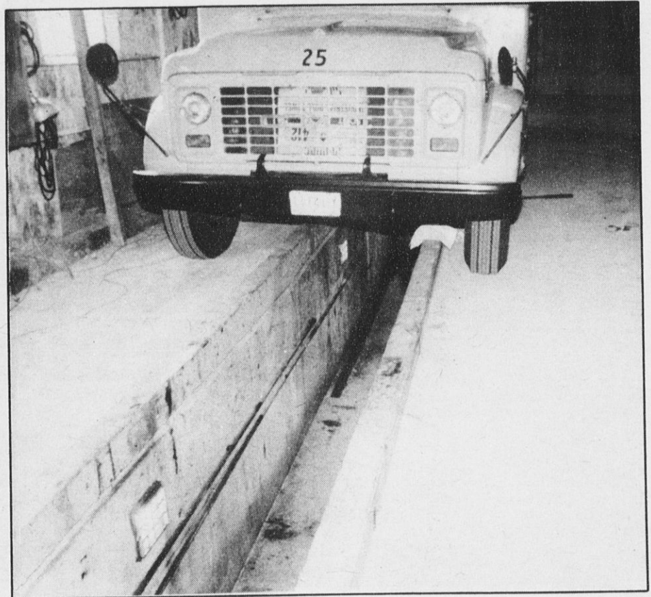
THE COST OF A RAILING for this vehicle service pit is re-imbursable by the state, according to Region III Health and Safety Specialist Linda Siccardi.
