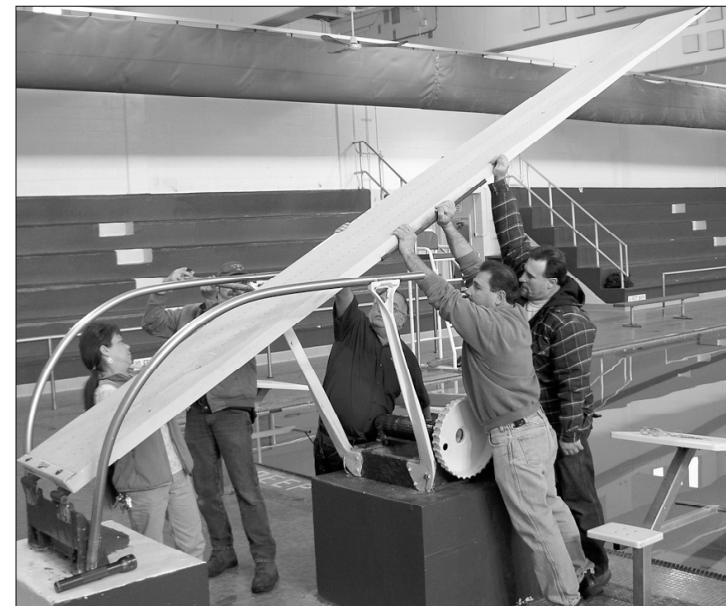
Sometimes it takes teamwork to set up for a function at school. Here, custodians and maintenance workers install the diving board for the Connetquot swim team.
