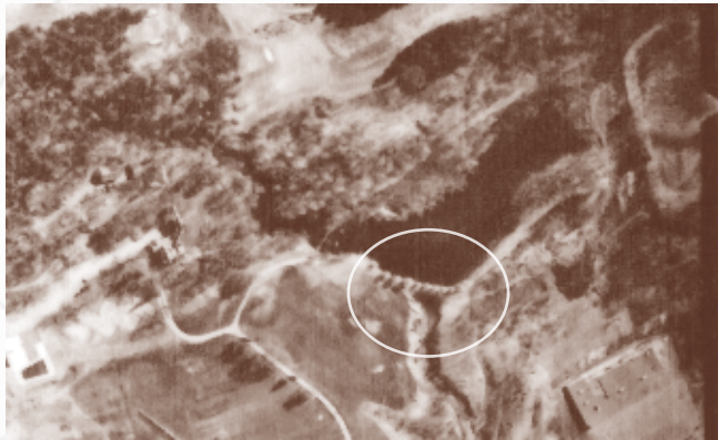
This 1962 photo from the University Archives shows the kuyl at the Albany Country Club (ACC). The wooden dam is circled.
