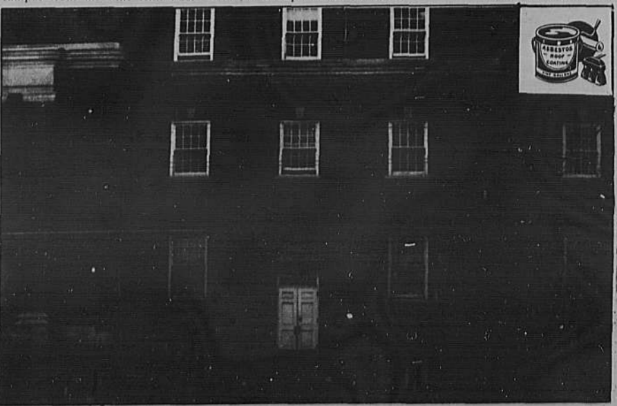
Richardson Hall has been cited for asbestos problems. The substance is considered very dangerous.
