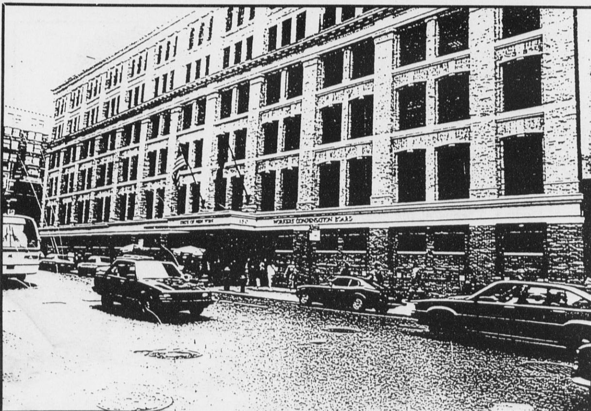
WORKERS' COMP BUILDING is a converted warehouse that, among other problems, is infested by rodents. CSEA's
