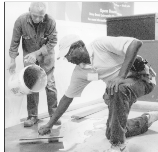
Plumber John Traynor, left, and Claude Corpening spread floor-leveling material.
