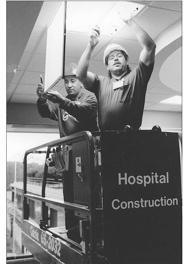
Ray Santiago, right, and Victor Perez, left, install light fixtures.
