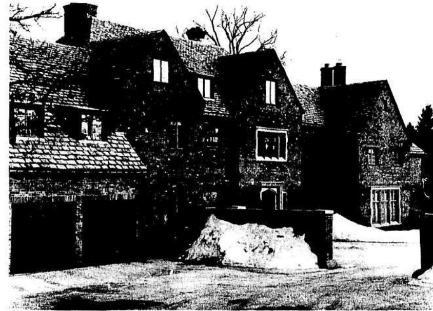
This is the $200,000 house provided for the State Education Commissioner Nyquist. However, Nyquist does not live in it; SUNYA President Louis Benezet does.
