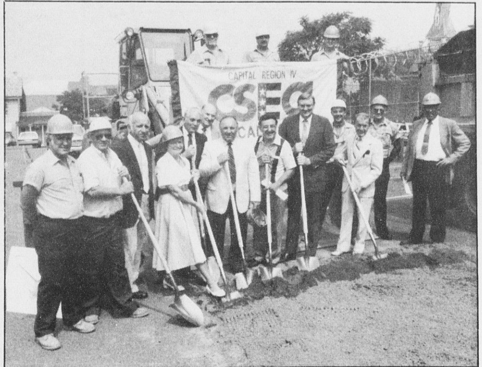
WORKING TOGETHER at the groundbreaking for the new addition to the Schenectady County Jail are both CSEA members, who are doing some of the work, and county officials. Third from left is Local 847 President Frank Tomecko, and at center is Engineering and Public Works Unit President Lou Altieri.
