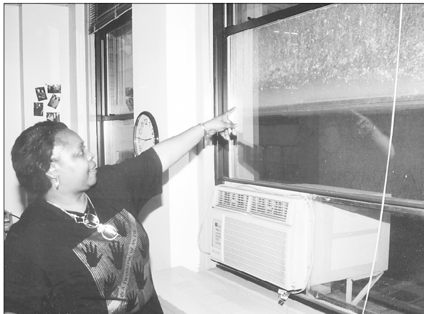
CSEA member Barbara Schoates points to some debris that remains on office windows since Sept. 11.
