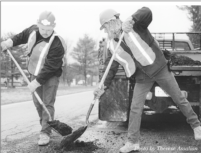
CSEA Clifton Park Town Unit members Ken Howland and Laurie Miller take part in a DPW rite of spring, filling pot holes along a road in the Capital Region.
