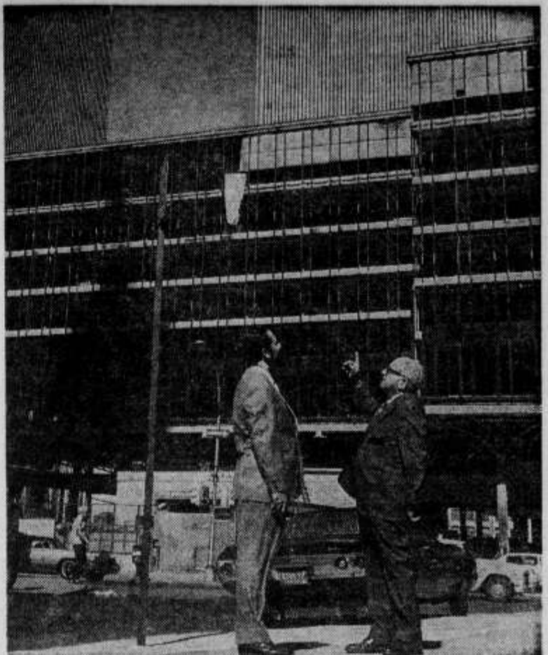
An on-the-scene inspection of the World Trade Center site to discuss fire safety precautions for State employees who will be assigned office space there, was conducted last week by Solomon Bendet, right, president of the New York City chapter, CSEA, and Frank Palumbo, vice-president of the International Association of Fire Fighters.
