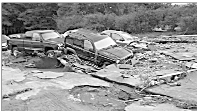
Flooding devastated highways much like this one in Sullivan County.
