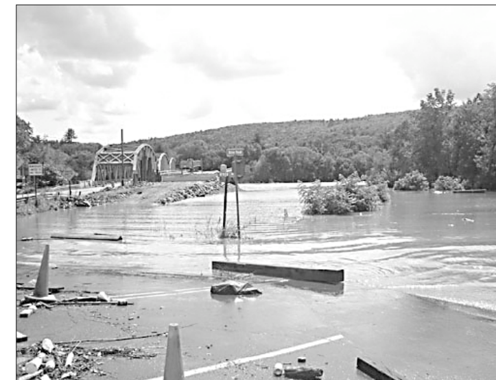
In a scene typical across a dozen New York counties, a roadway disappears into a flood-swollen creek in Sullivan County.
