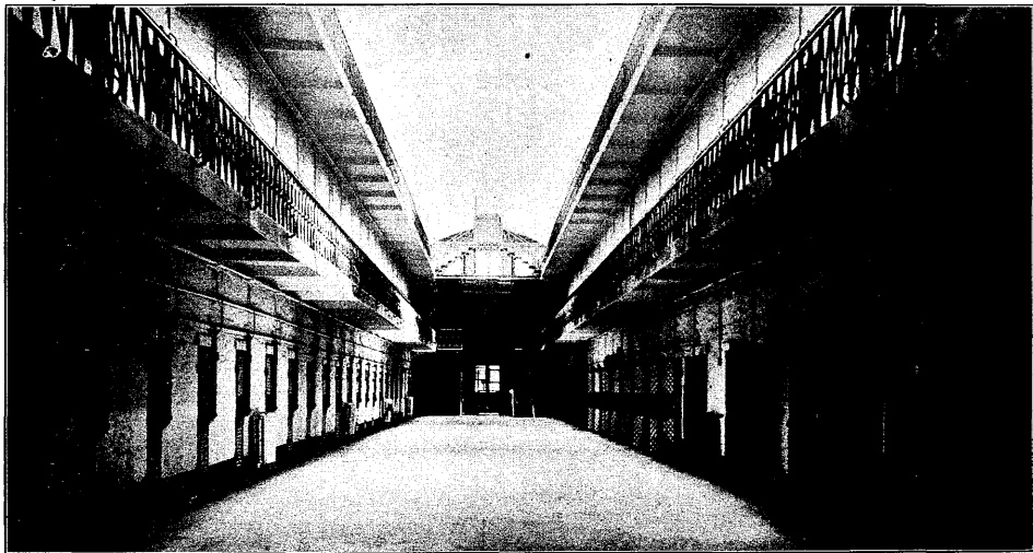
THE INTERIOR OF THE NORTH WING, OR PRISON SECTION, OF CORRECTIONAL HOSPITAL FOR FEMALES ON WELFARE ISLAND
