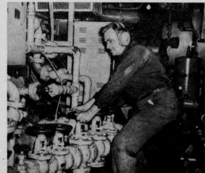
The deafening noise of the tug's engines doesn't show up in the photo, but engineer Al ReSavage wears protective earphones as he regulates the valves below deck in the engine room.
