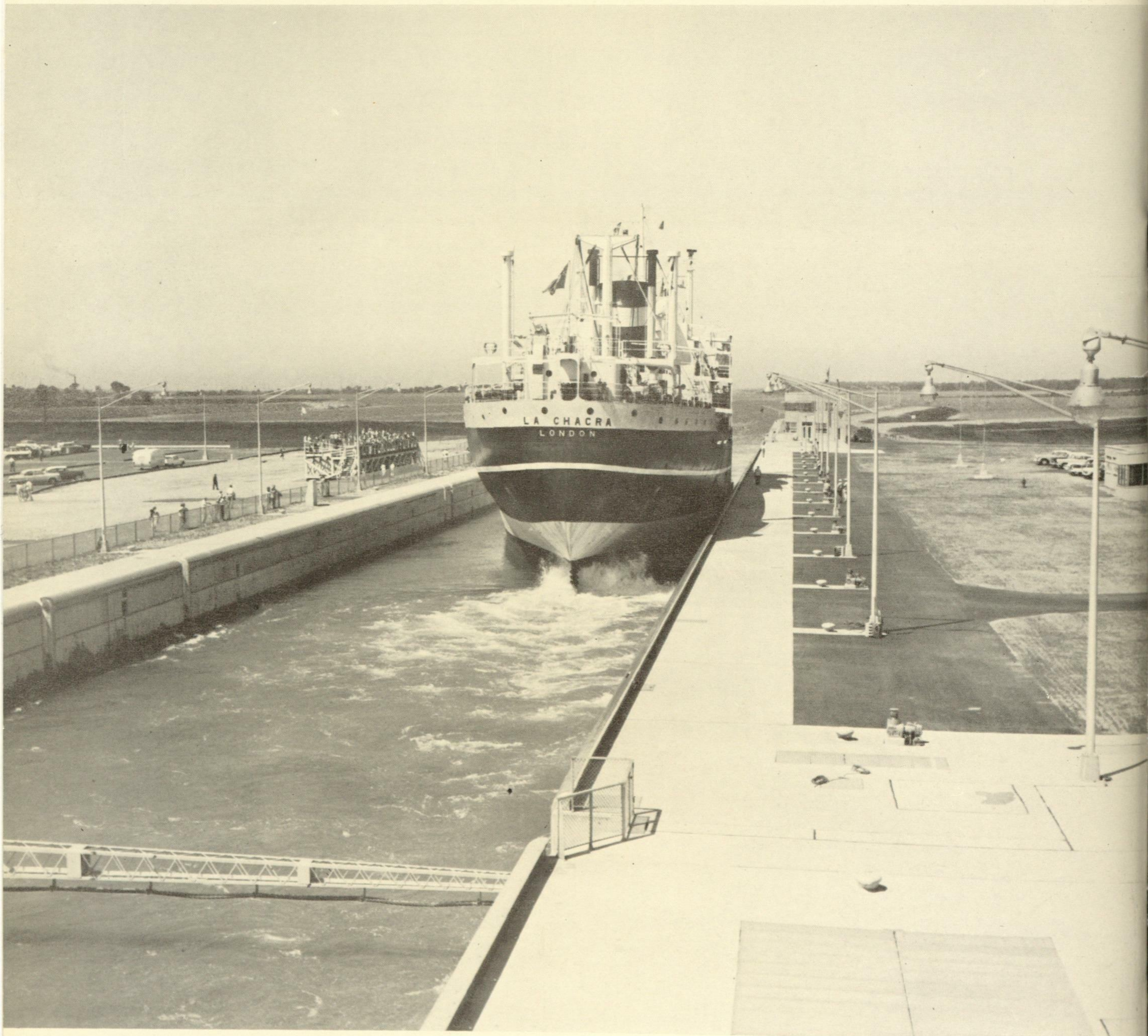
Eisenhower Lock at the southern end of the Wiley-Dondero ship canal near Massena, N. Y. lifts or lowers St. Lawrence Seaway traffic 42 feet into or from the power pool. Facilities are provided to enable visitors to watch locking operations. Above: a ship out of London, on its way to the Great Lakes, leaves the lock.
