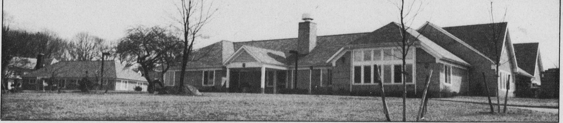
One of the brand new intensive care units on the grounds of the former Staten Island Development Center.
