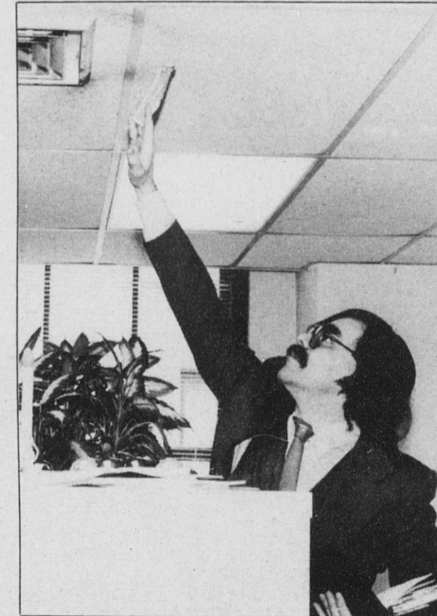
IN DESCRIBING THE VENTILATION in the Yonkers DSS building, CSEA Collective Bargaining Specialist Al Sundmark said, "There is none."
