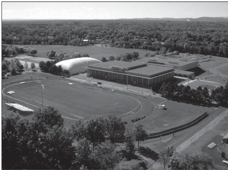
Albany's athletic facilities include University Field, University Gym, the RACC, and the Bubble.
