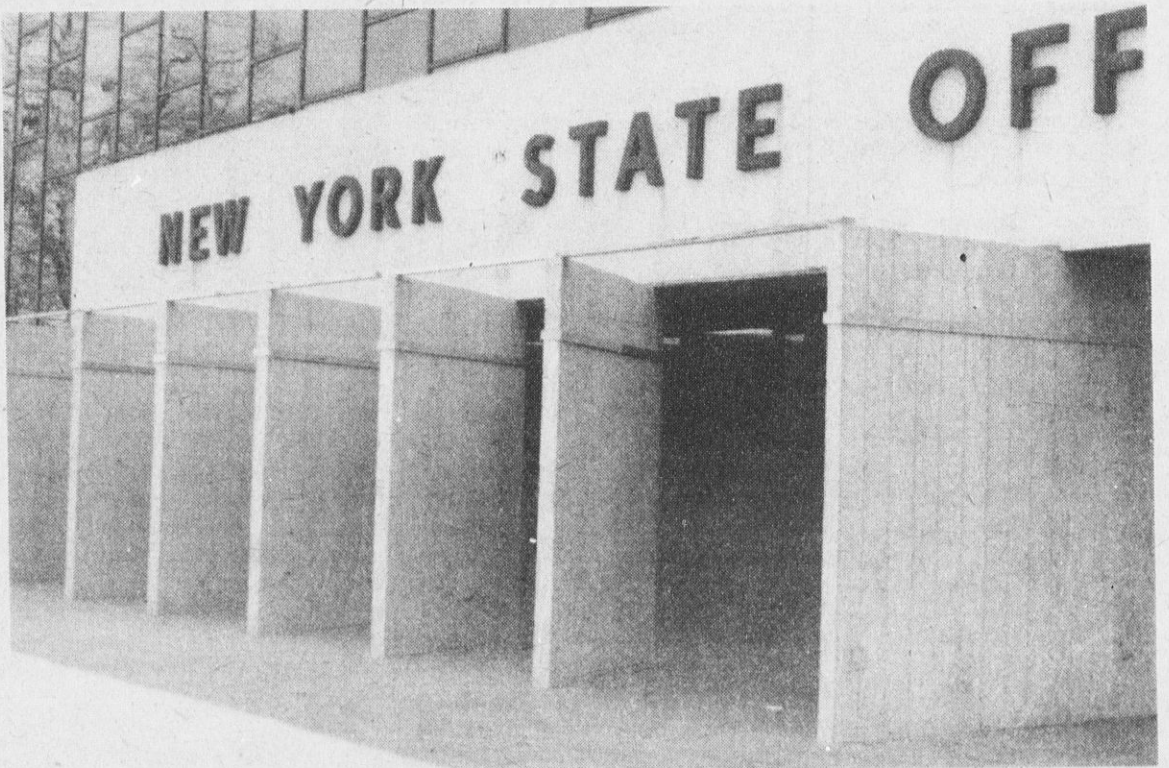
TEMPORARY WIND BREAKS were constructed outside and inside the front doors of the State Office Building in Hauppauge when cold air entering the building forced many employees to work in coats, hats and gloves. Hauppauge State Office Building Local 016 President John Madion, above, stands by the windbreak inside the building.
