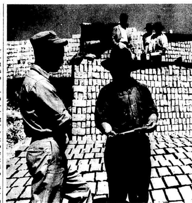
James Welcome, a graduate of the University of Illinois, is a member of a community development project, in Colombia. Here he supervises brick-making, a project the local people have undertaken with the help of the Volunteers.
