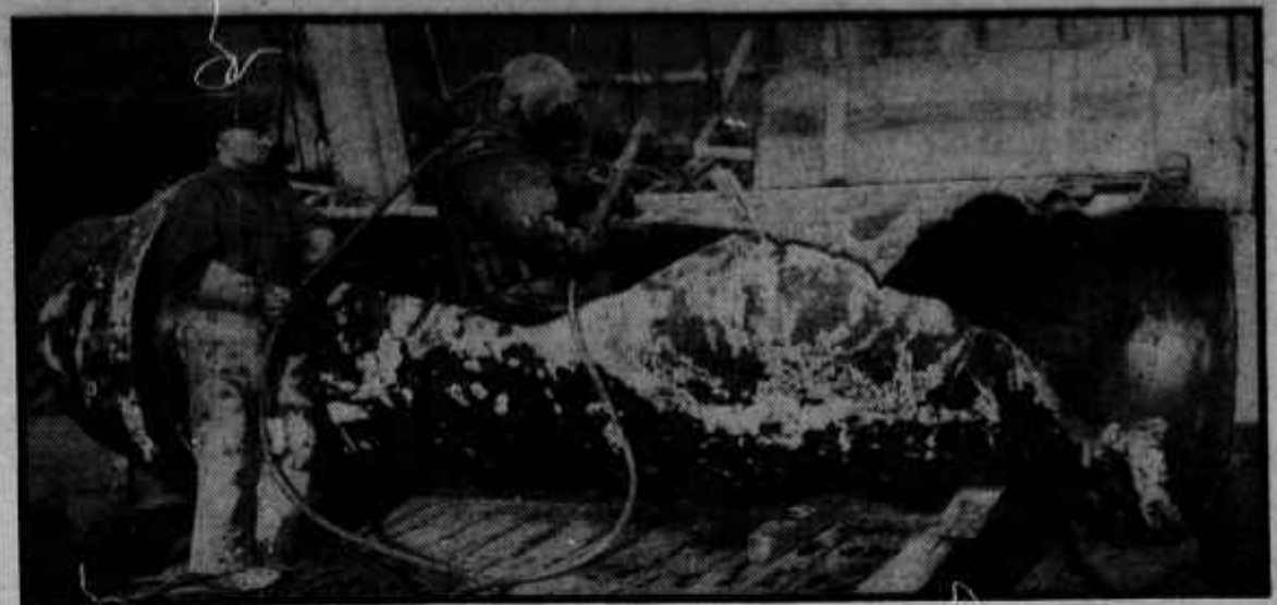
You'd be amazed at the kind of people who work for the Government. Here, for example, we dug up a diver (no pun intended), who works for New York City's Department of Water Supply, Gas, and Electricity. He has regular status, and all that goes with it. We caught him on the waterfront, using an electric torch to do a repair job. The electric wire and cutting gas are carried through the hose, shows below the diver's right hand. He sure deserves that raise, Mr. Mayor!
