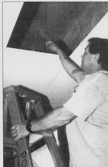
CSEA member Mike Bard, a certified pool operator, cleans the pool at Valley Central High School. At right Bard shows how he checks stainless steel wires that hold up the ceiling.
