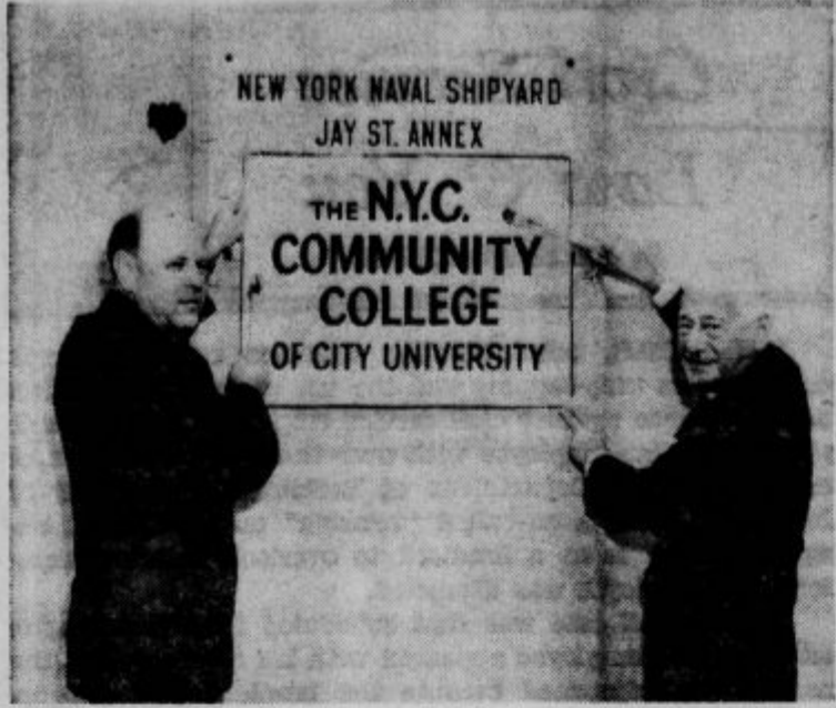
COLLEGE — Dr. Murray H. Block, left, acting president of the New York City Community College of City University, and Brooklyn Borough President Abe Stark proudly affix the sign of the new owners on the New York Naval Shipyard, Jay Street Annex. The largest community college in the City and the State acquired the eight-story brick and concrete building at Jay and High Streets with the final signing of the deed by Mayor Robert F. Wagner.
