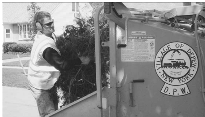
Greg Urbanski operates sanitary sewer cleaning equipment on a Depew village street. The high quality of services is jeopardized if the village is dissolved.
