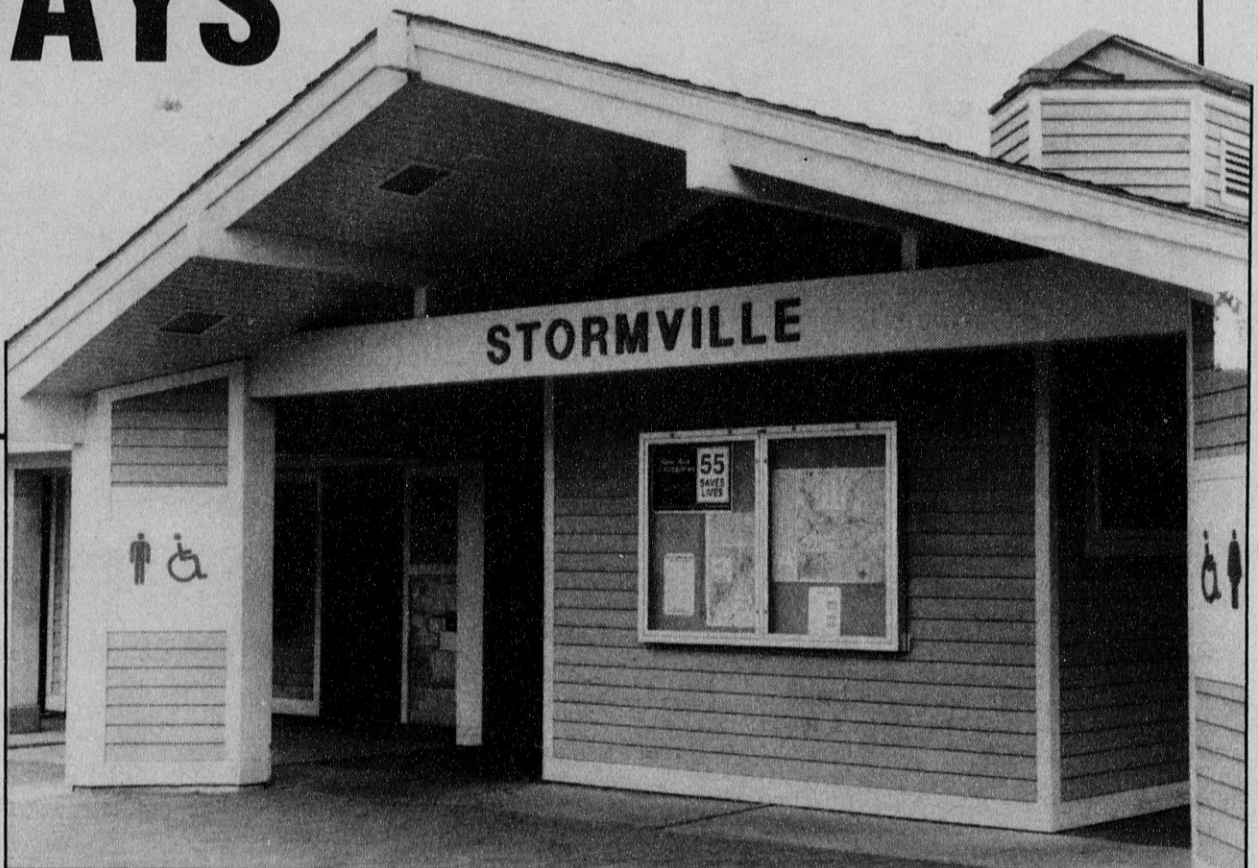
THIS STORMVILLE REST AREA along I-84 appears clean and inviting after state DOT employees cleaned it up. But over the next 24 hours it will be trashed up again. Workers often find health hazards inside the building, in trash containers and scattered around the parking areas.
