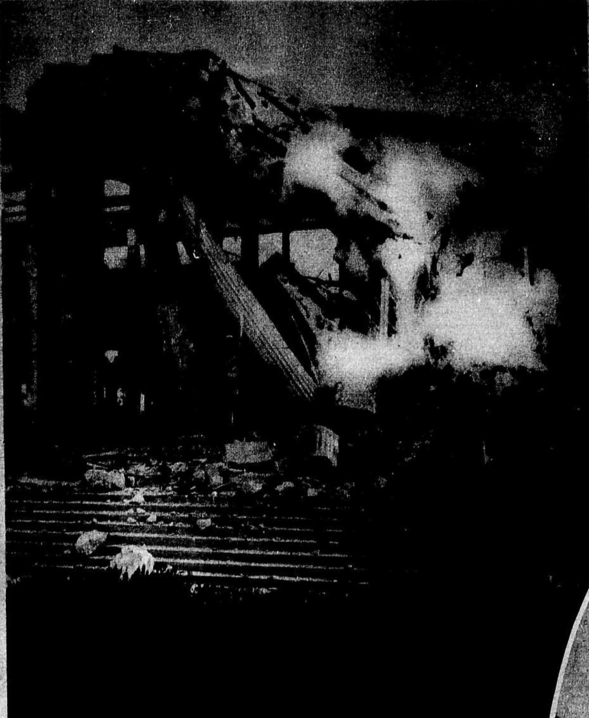
CONDEMNED FOLLOWING DAMAGE BY EARTHQUAKES , Pasadena (Calif.) Junior College buildings were demolished to make way for new and earthquake-proof structures. This remarkable action photo shows the front of the main building crashing after the key pillar was removed.
